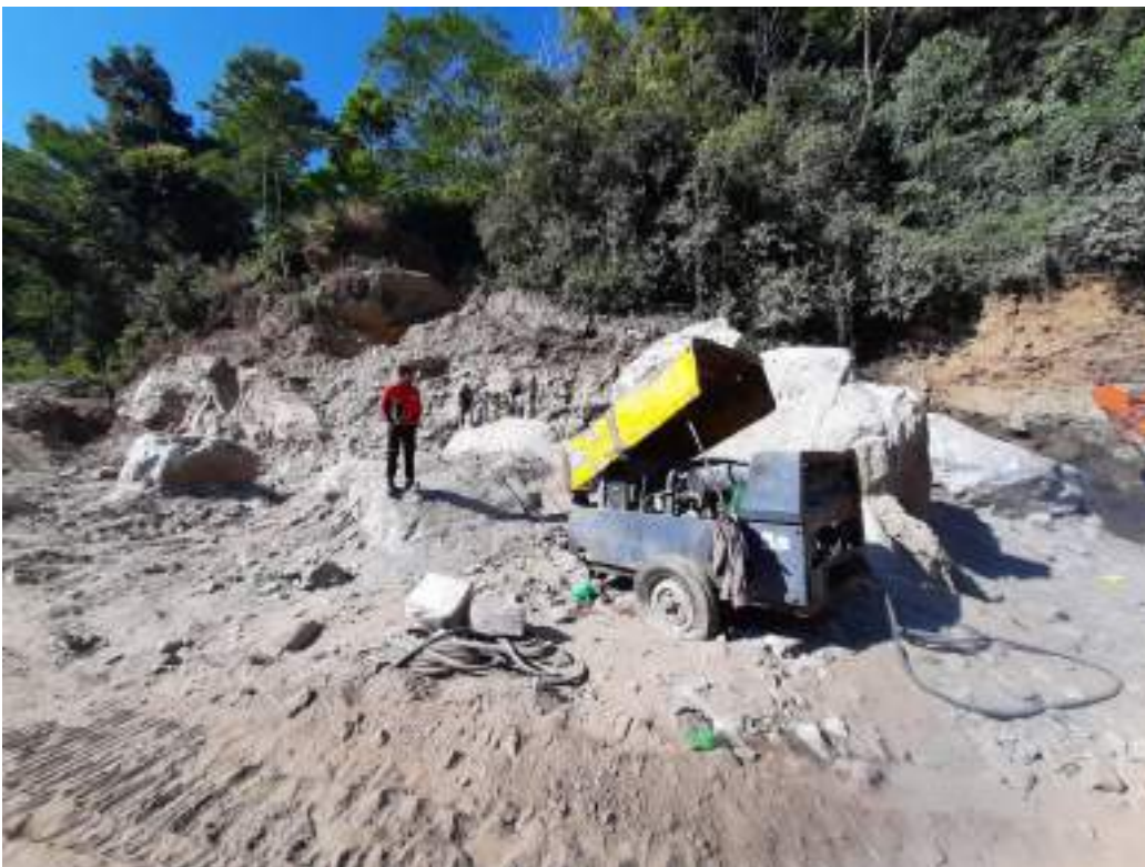
Figure 4-9: Compressor used for drilling process
