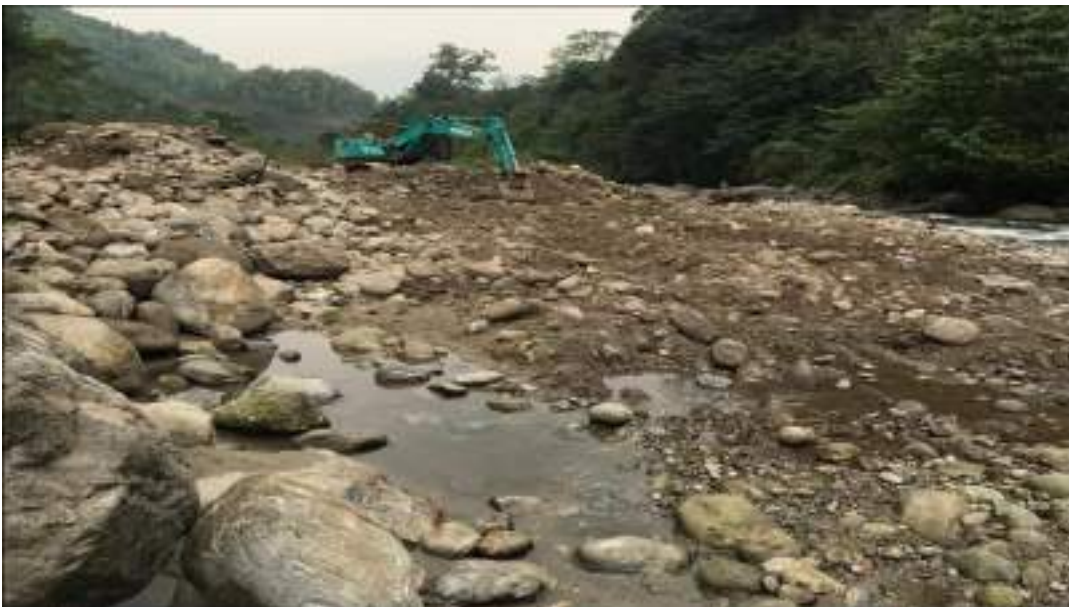
Figure 4-16 Collection of Construction Material at the Powerhouse Area
