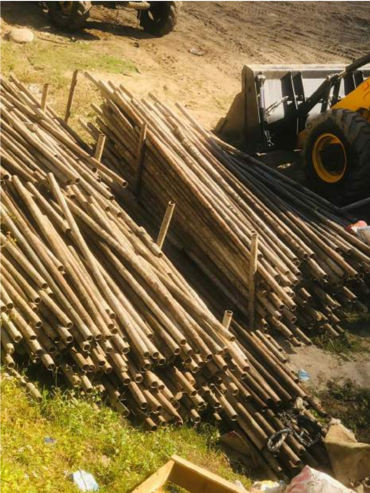
Photograph 10: Pipes stock for multi-purpose use.
