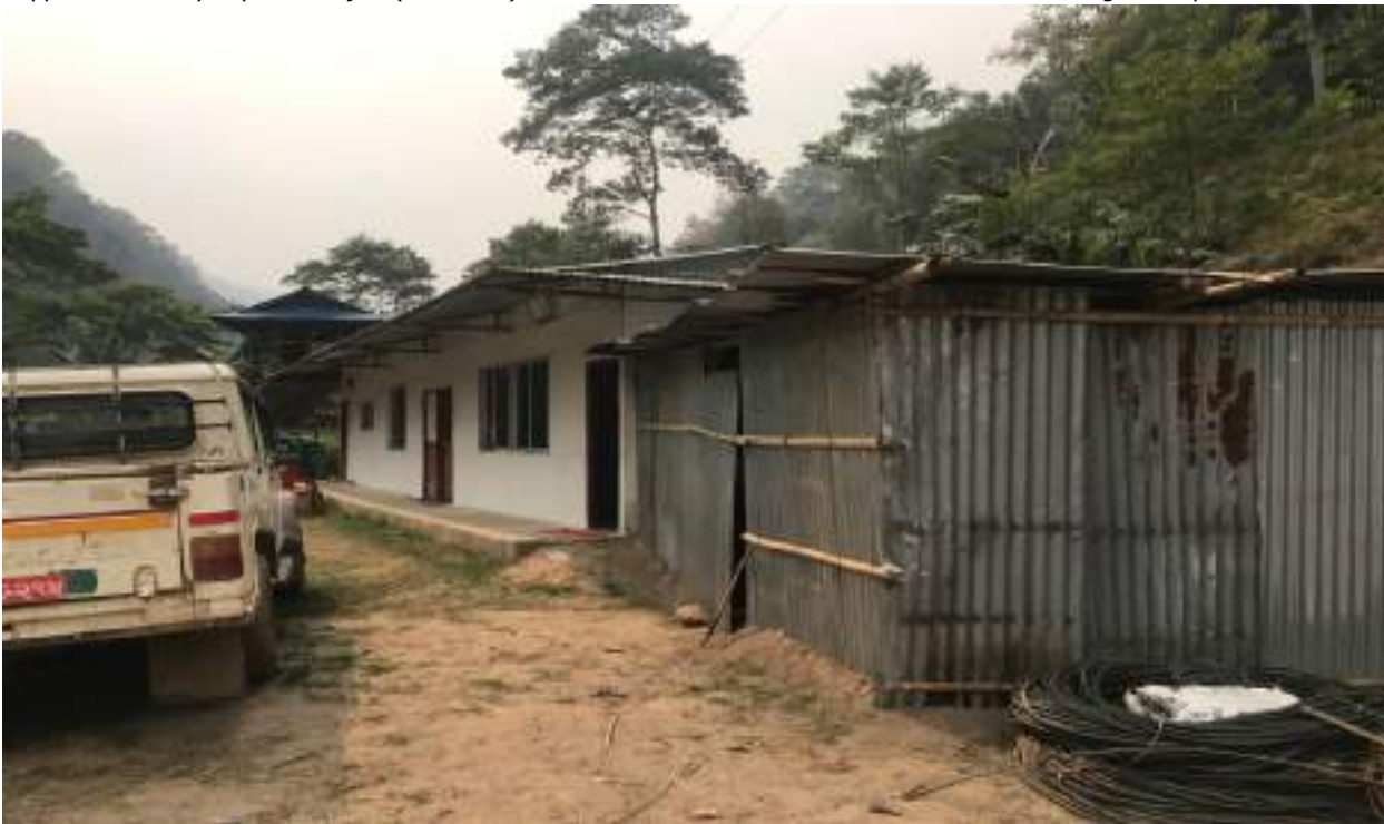
Figure 4-2 Constructed Camp near Powerhouse Area of UIHPP
