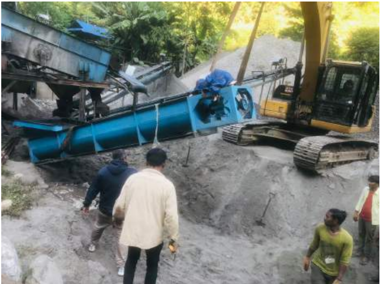
Photograph 8: Installation of Crusher plant
