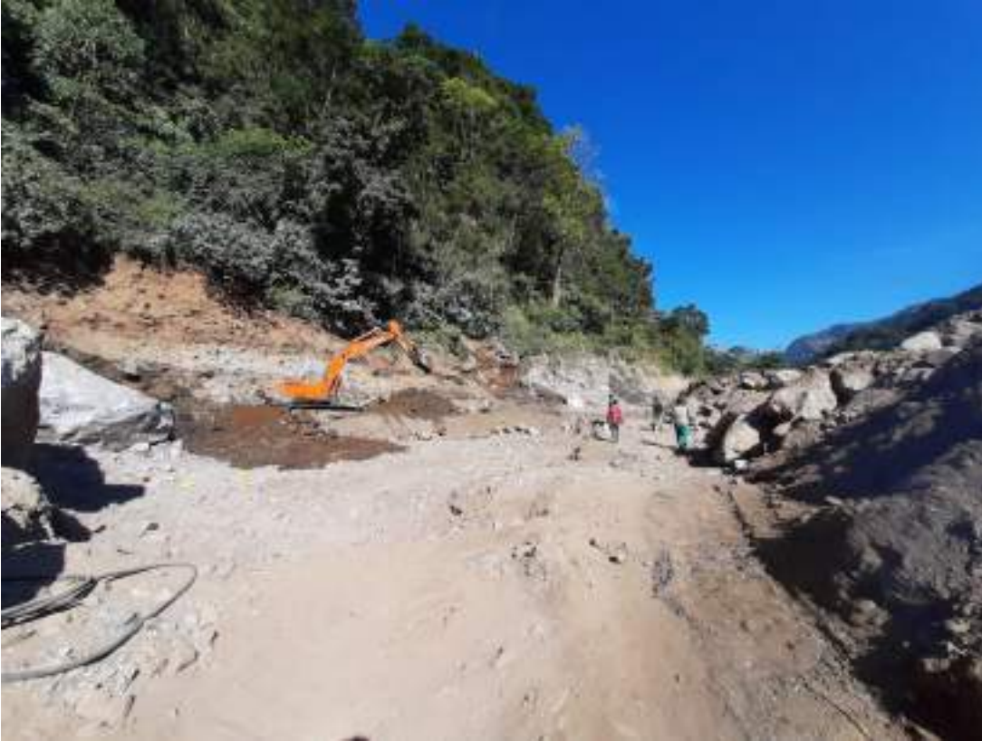
Figure 4-8 Site clearance works at Intake and Settling Basin Area-1
