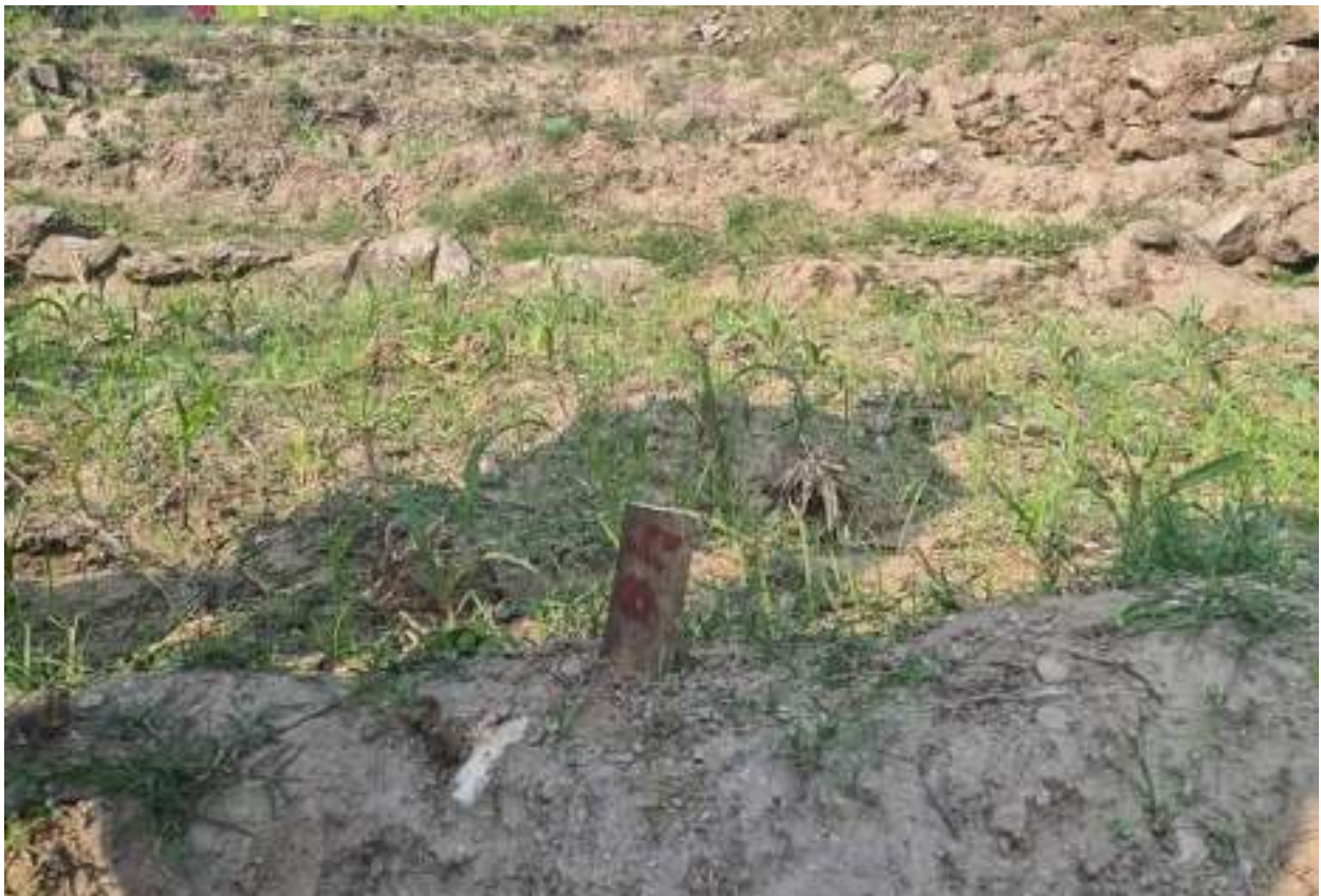
Photograph 5 : Layout Works of Pipe Alignment
