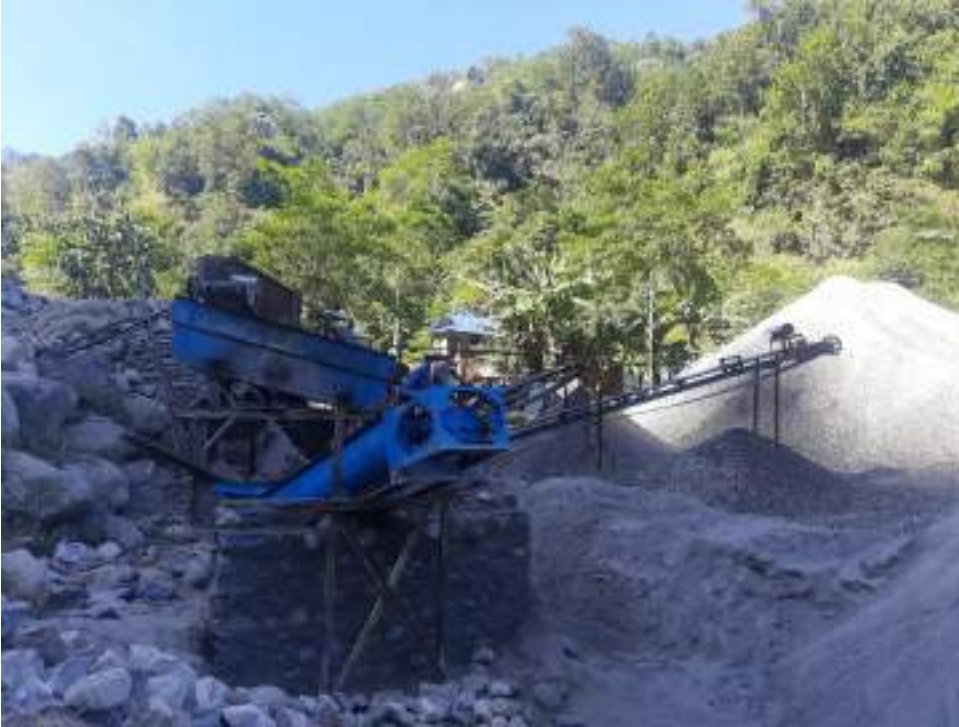
Figure 4-5 Crusher plant Area
