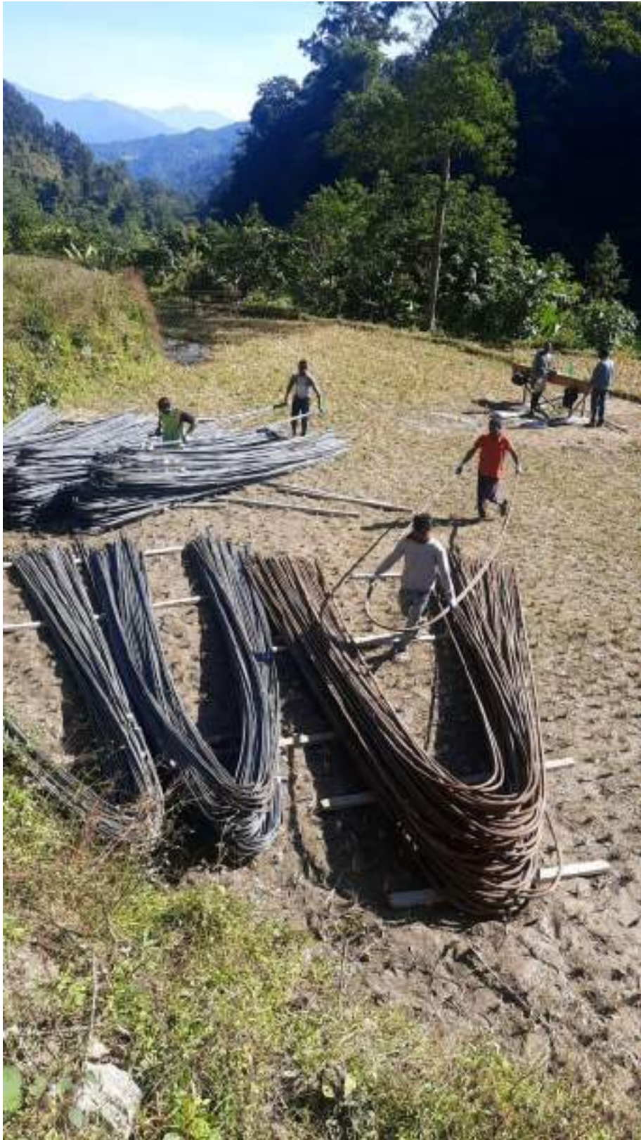
Photograph 11: Bar bending work under process
