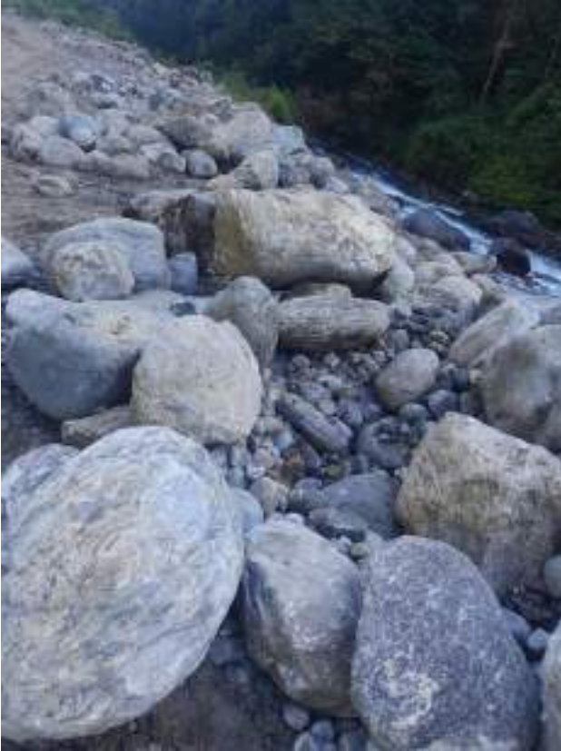
Figure 4-17 Collection of Quarry Material Near Powerhouse Area
