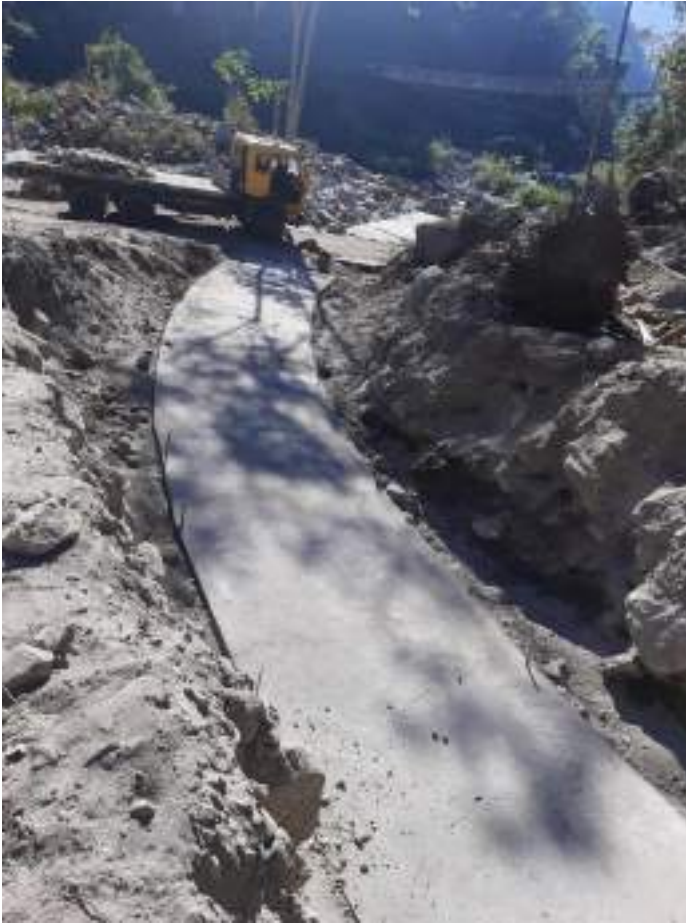
Figure 4-10: PCC work for excavated approach canal.
