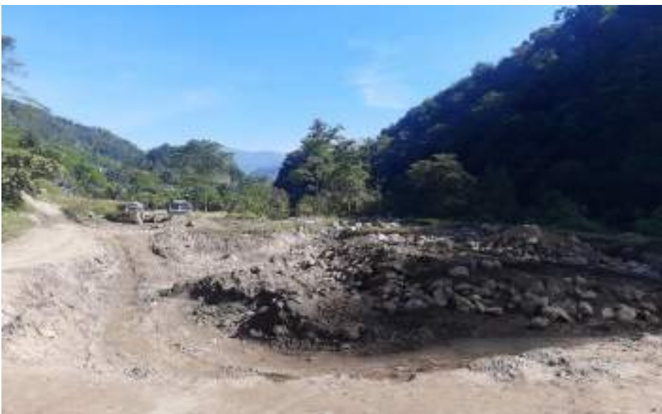
Figure 4-7: Excavation work at powerhouse area
