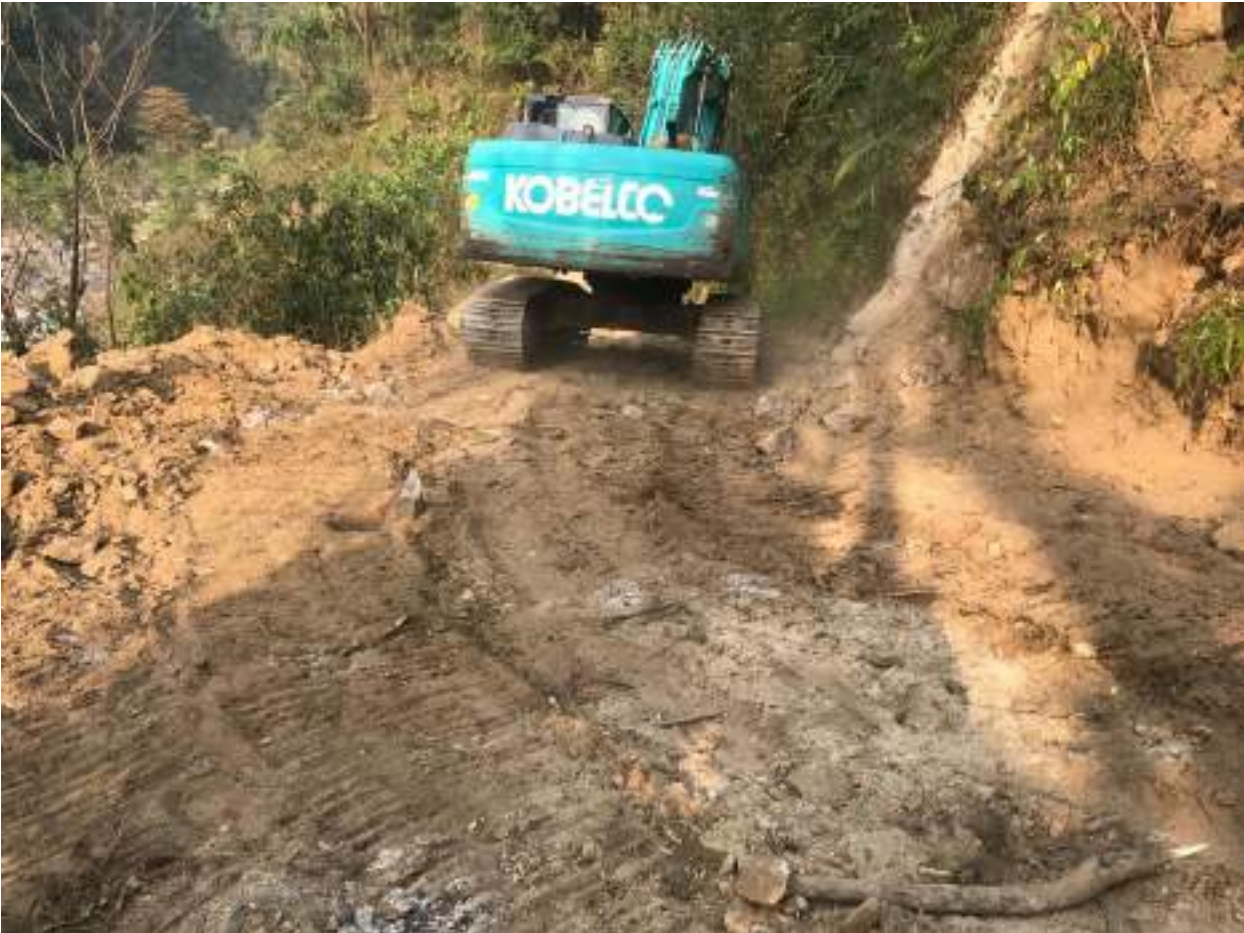
Figure 4-13: Access Road towards Gothe bazar to Headworks Area-3
