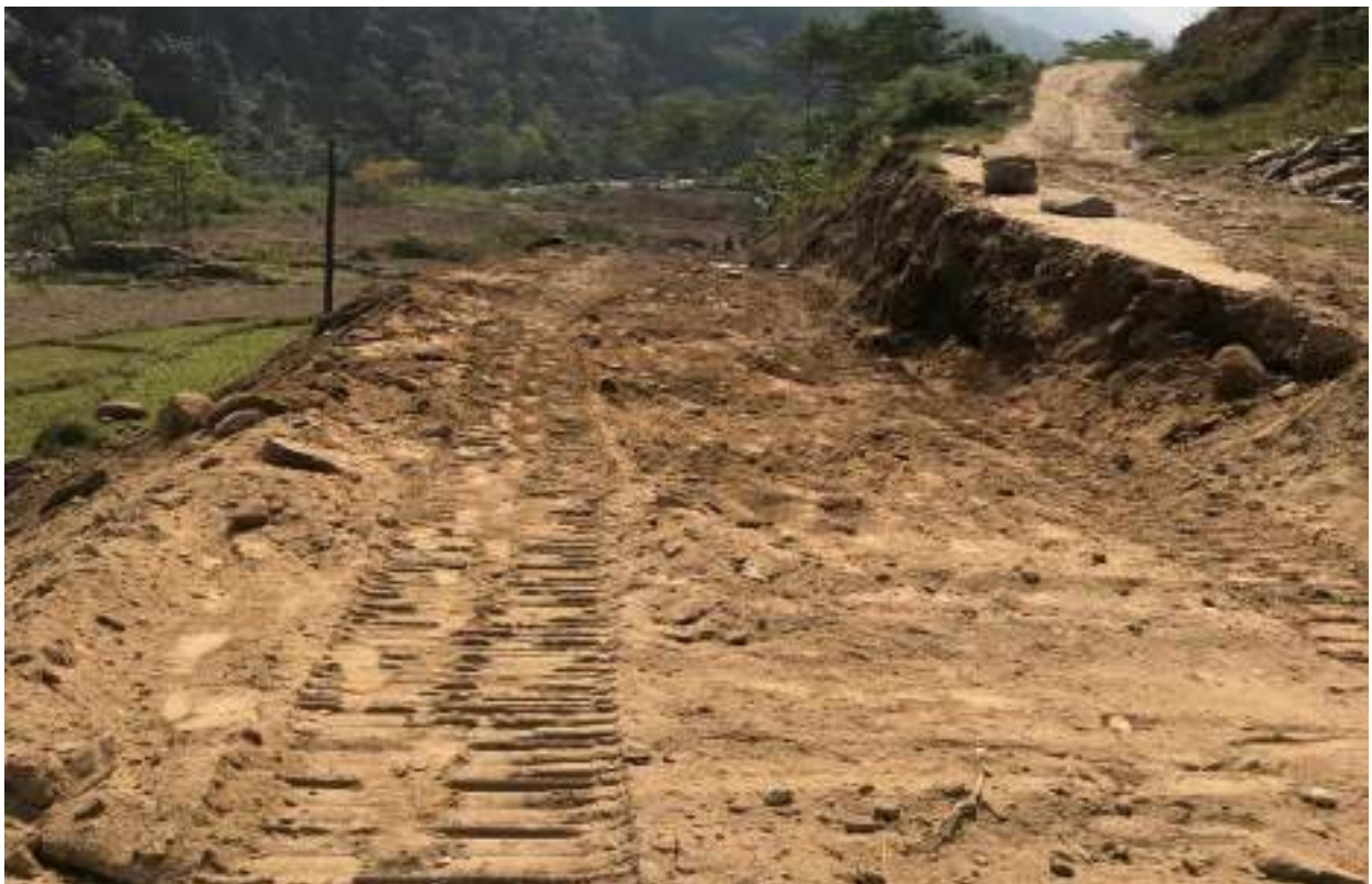
Photograph 9: Road towards Powerhouse Area and Camp house
