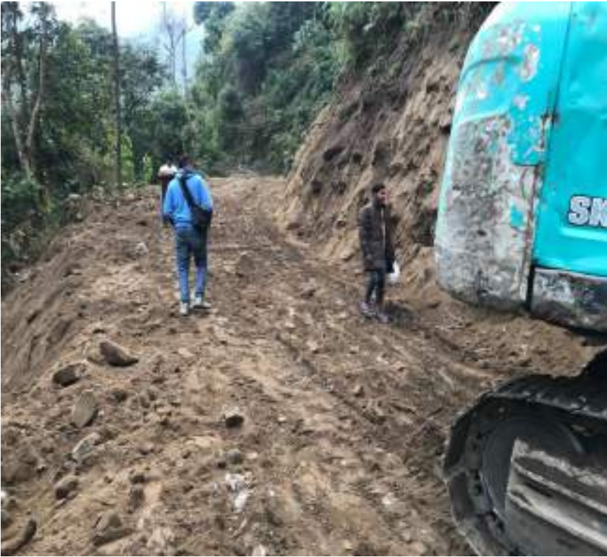
Figure 4-11: Access Road towards Gothe bazar to Headworks Area-1
