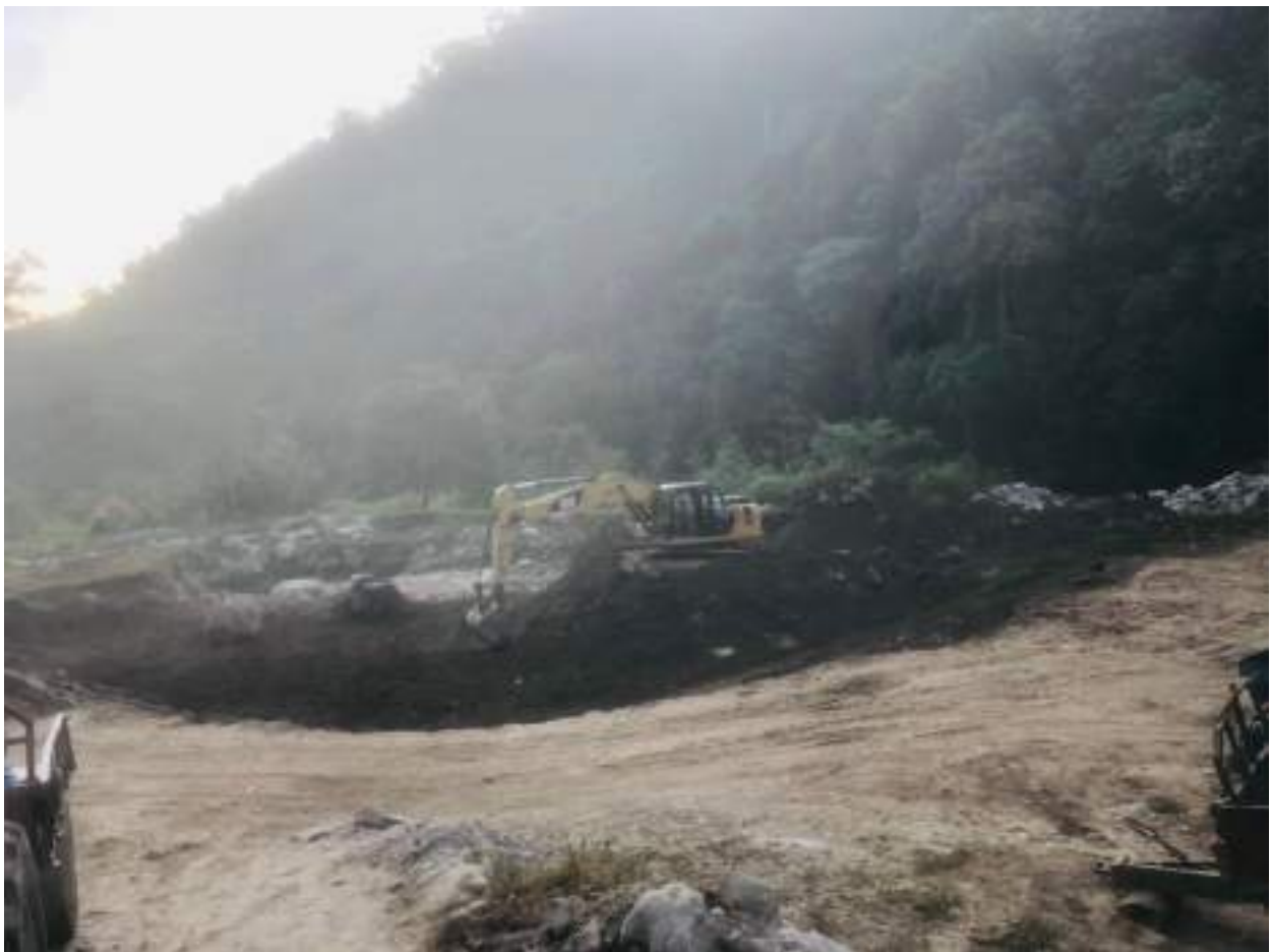
Photograph 13: Excavation work in Powerhouse area under process
