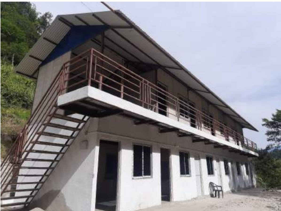
Figure 4-3 Newly constructed Camp house at Powerhouse Area
