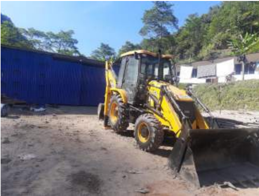
Figure 4-6: Newly purchased backhoe loader at site.
