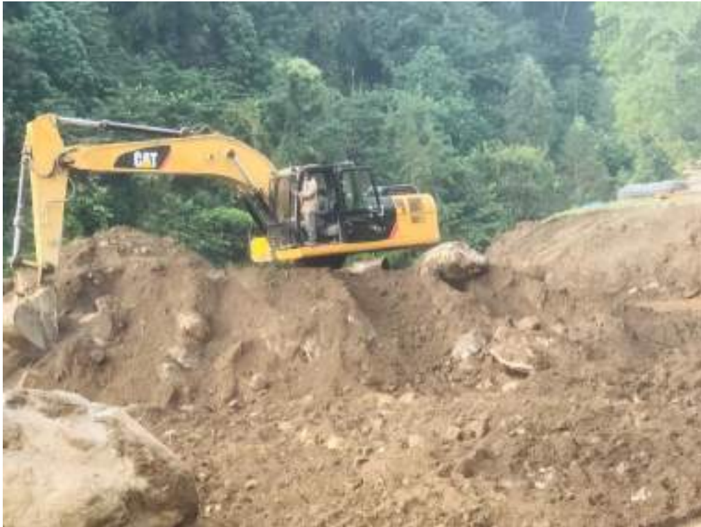
Photograph 12: Excavation work in Powerhouse area under process
