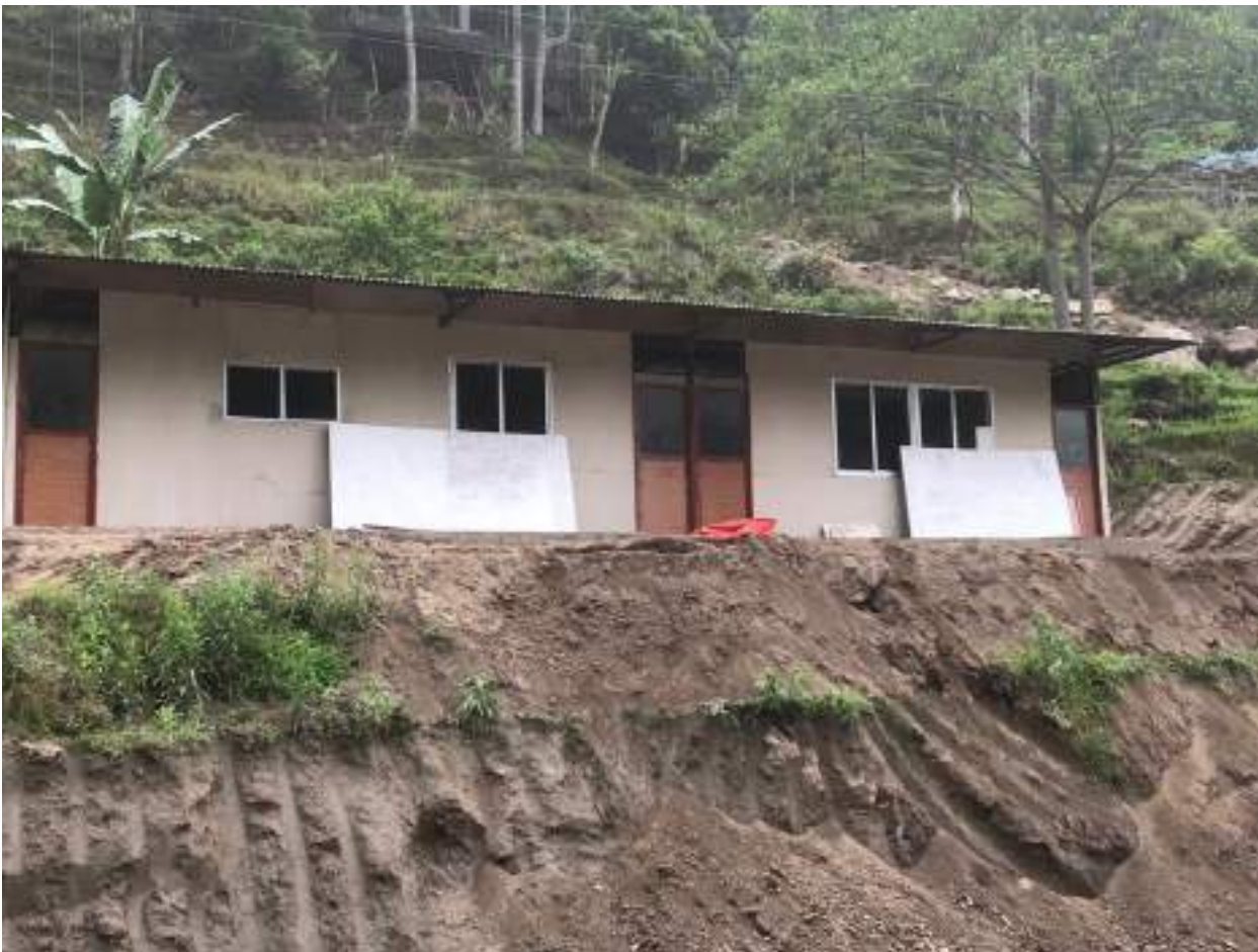
Figure 4-1 Construction of Camps at Powerhouse Area
