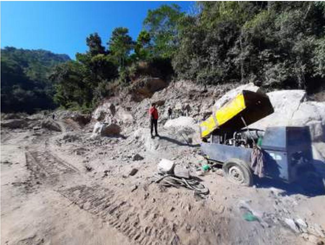
Figure 4-9 Site clearance works at Intake and Settling Basin Area
