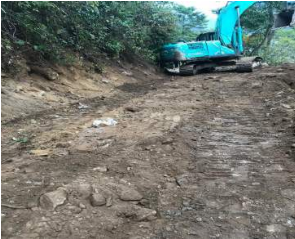
Figure 4-12: Access Road towards Gothe bazar to Headworks Area-2
